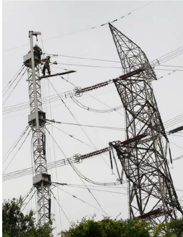
Linesmen are connecting conductors on a 70-feet high temporary mast. The construction of a temporary mast takes a little over 10 days, which is over 10 times faster than repairing a damaged tower
