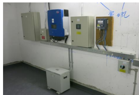
RE system equipment
