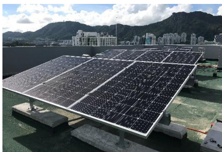
PV panel and structure
