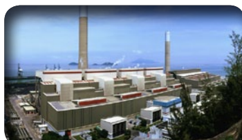
Low NO x burners at Castle Peak Power Station
