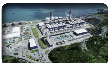
Natural gas-fired generation at Black Point Power Station
