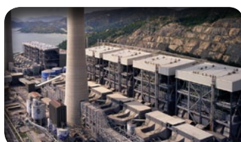
Emissions Control Equipment at Castle Peak Power Station
