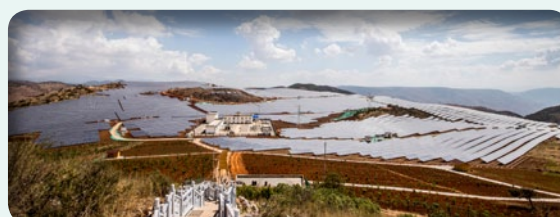
Xicun Solar Plant, Yunnan, China
