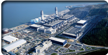
Black Point Power Station which uses natural gas for electricity generation
