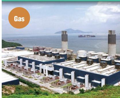
8 x High Efficiency Combined Cycle Gas Turbines
