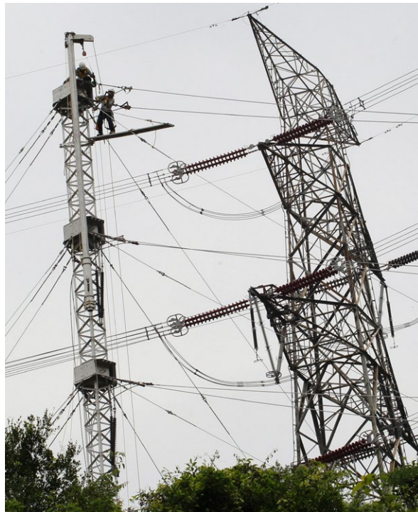
Linesmen are connecting conductors on a 70-feet high temporary mast. The construction of a temporary mast takes a little over 10 days, which is over 10 times faster than repairing a damaged tower.
