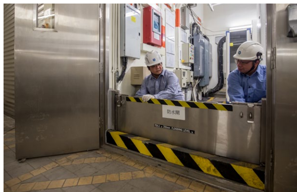
Flood-prone transmission and distribution substations are equipped with flood gates.
